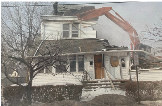
2004 demolition of the original church, which had become a private home
